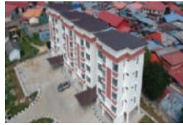
Hospital Semporna Quarters, Sabah
