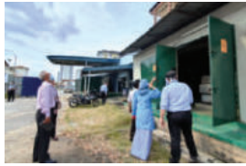
Chiller Room Hospital Tengku Ampuan Rahimah, Klang
